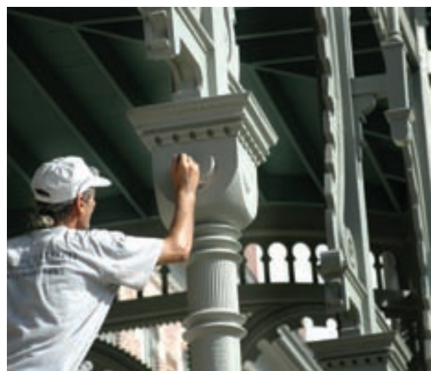
Painting Plant Hall's crescent moons a metallic silver is one element of restoring the building to its original color scheme.
