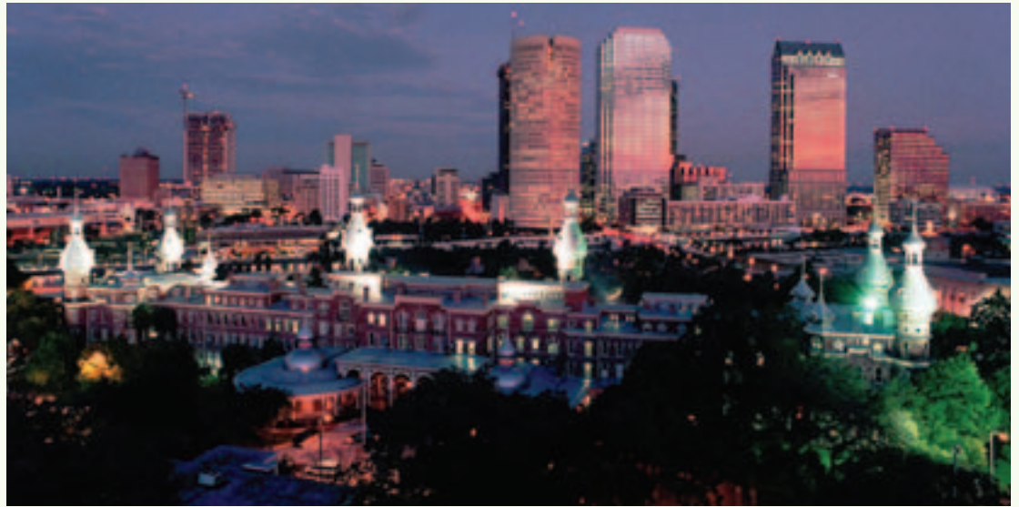
The Chiselers were instrumental in acquiring funding for a roof-line reconstruction of the Plant Hall roof in the early 1990s.
